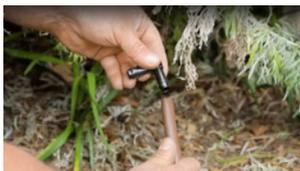
Use **13mm Elbow** or **Tee** fittings to join a new section of tube.
