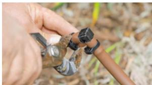
Secure the fittings in place using **13mm Locking Clamps**.
