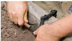
If there is some distance between your water source and the Drip Eze, connect it using **13mm poly pipe**.
